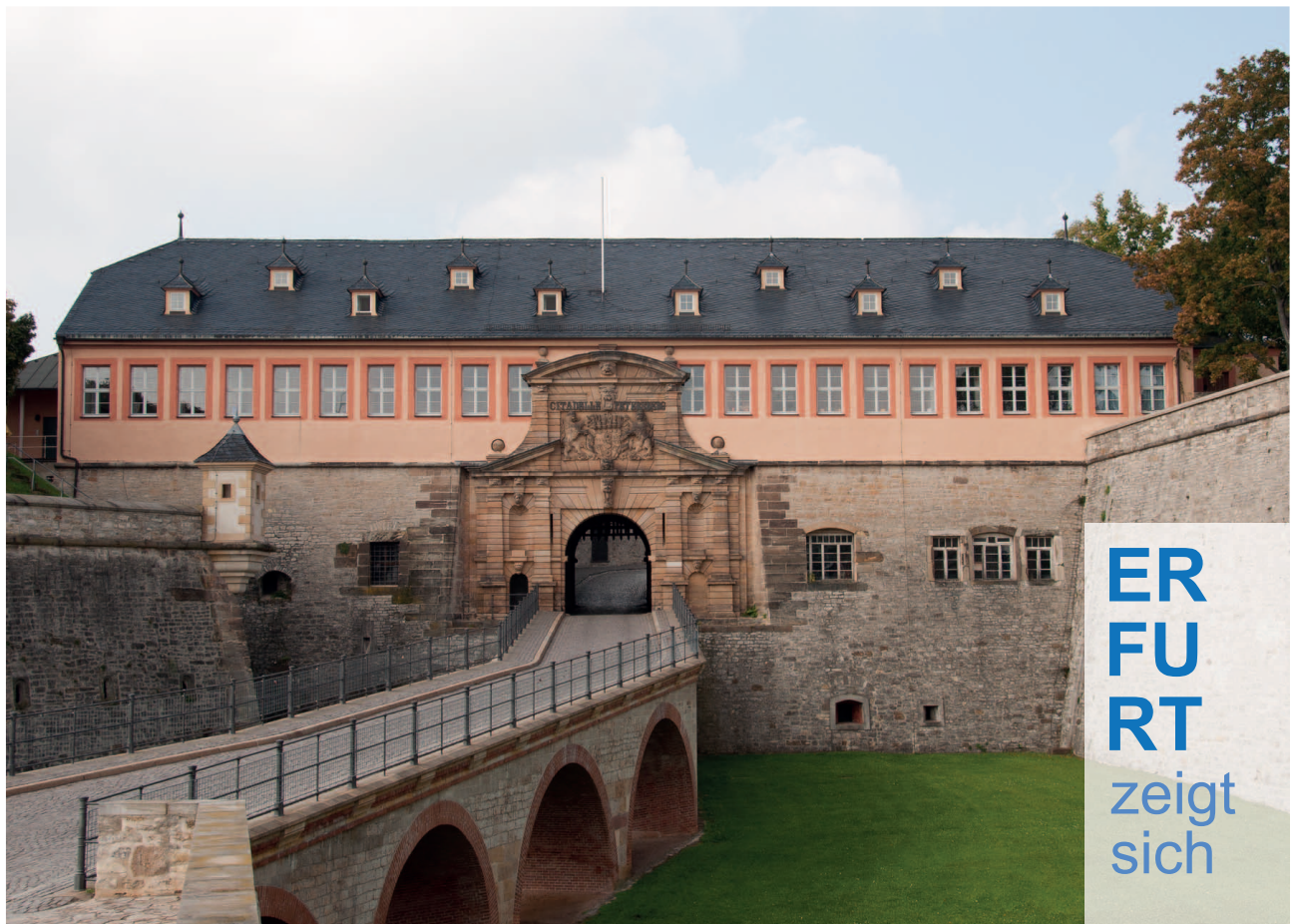
21 Kommandantenhaus - Commander's House
