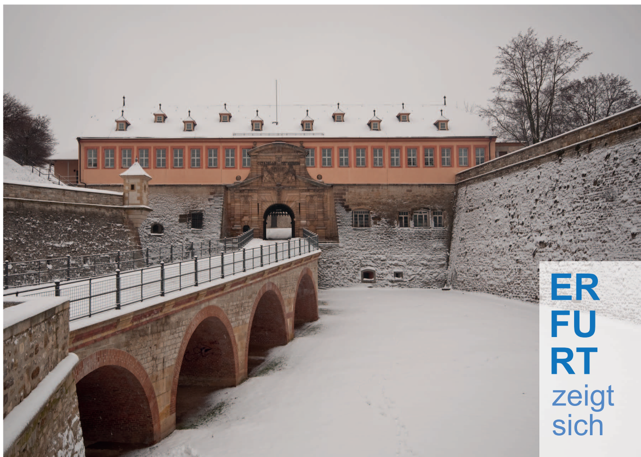
22 Kommandantenhaus - Commander's House
